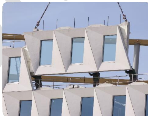
Figure 6.2 - Precast Frame
